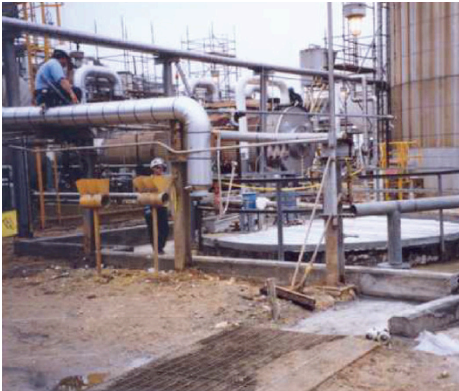
4. Completed sulfur pit from a ground view
