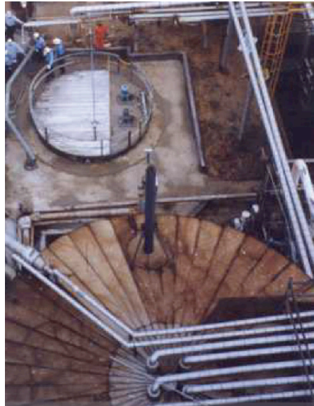
5. Completed sulfur pit from an aerial view
